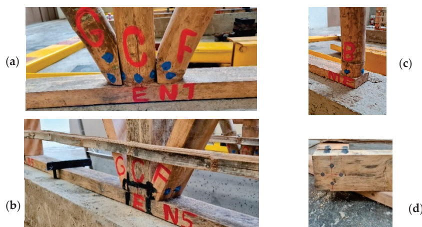
Figure 8. (a) An example of a steel nail connection at the central joint of a bahareque wall with a guadua skeleton (vertical element and two braces) (Blue points indicate the position of the steel nails); (b) an example of a steel nail connection at the central joint of a bahareque wall with a wooden skeleton (vertical element and two braces); (c) an example of a connection between a guadua vertical element and a wooden sill beam; (d) an example of a connection between a wooden vertical element and a wooden sill beam.
