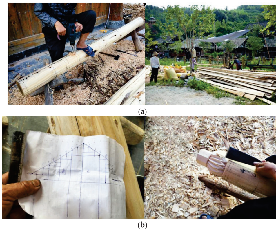
Figure 5. Traditional dwelling construction in Qiandongnan Xiaohuang Village. (a) Construction of traditional dwellings involves use of various woodworking tools, such as axes, chisels, planes and saws. (b) Simplified construction methods rely on direct carving and experiential knowledge of local artisans.
