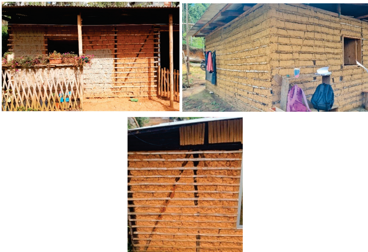
Figure 2. Bahareque dwellings with guadua strips located in the village of “La Estrella” near the municipality of Jamundí, in the Valle del Cauca Department, southwest Colombia.
