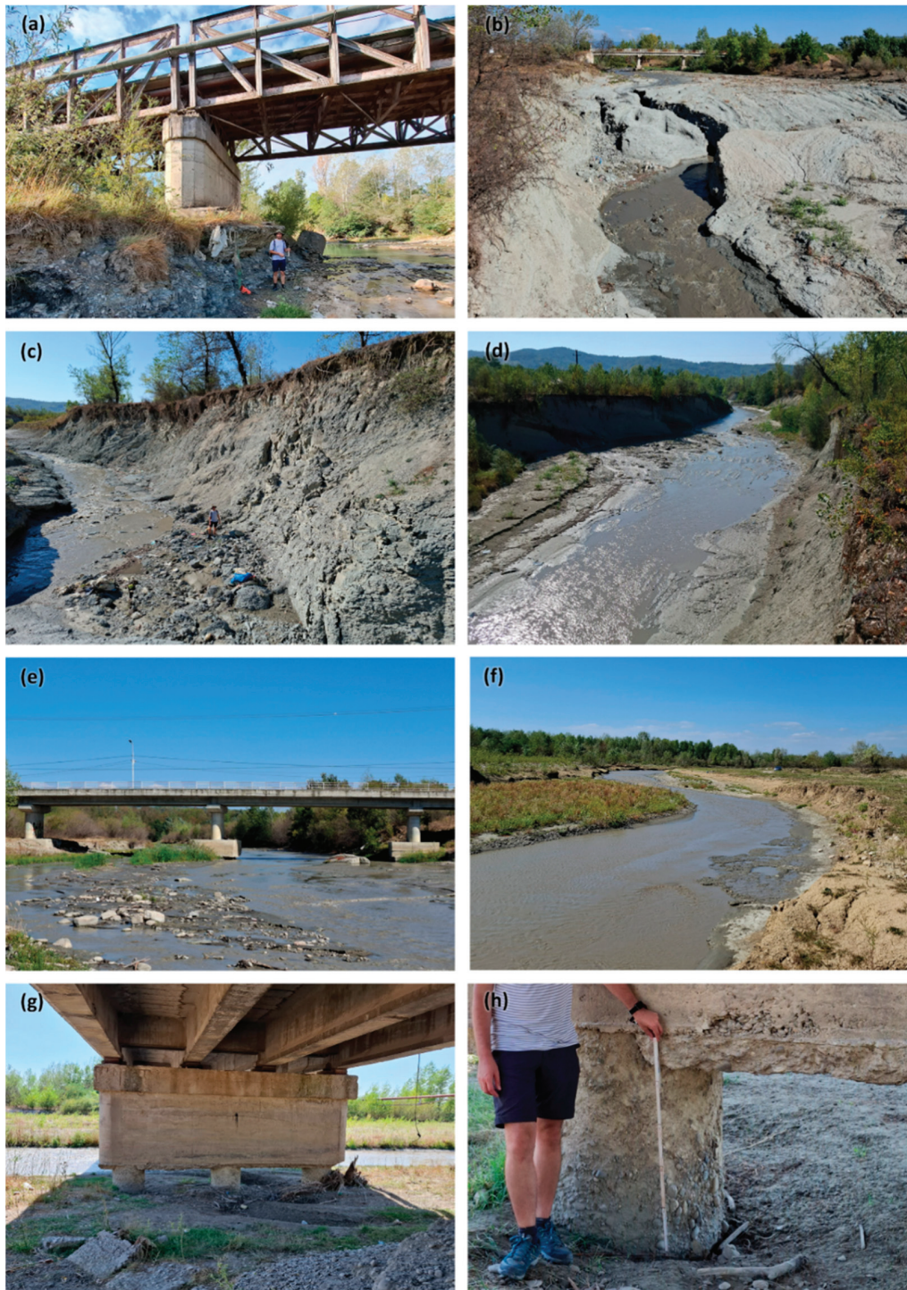
Figure 16. Observed riverbed incision and its impact on bridge structures along the studied Ialomița River reach. The images are ordered from north to south as follows: (a) bridge pier erosion near Fieni; (b–d) very intense riverbed incision in the Subcarpathian zone south to Pucioasa; (e) incision affecting 2 of 3 bridge piers on DC136B road near Brănești; (f) incision in the exploitation area of a former gravel pit (GP2 in Figure 15); (g) intense incision at bridge pier on DJ711B road at Băleni; (h) incision of over 1 m (length of the white ruler) at the base of the pillar. The riverbed has silted up due to the ongoing dredging of Lake Pucioasa.
