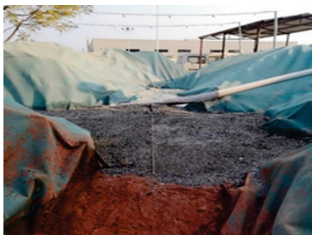
Figure 7. Second-stage sub-dam stacking.
