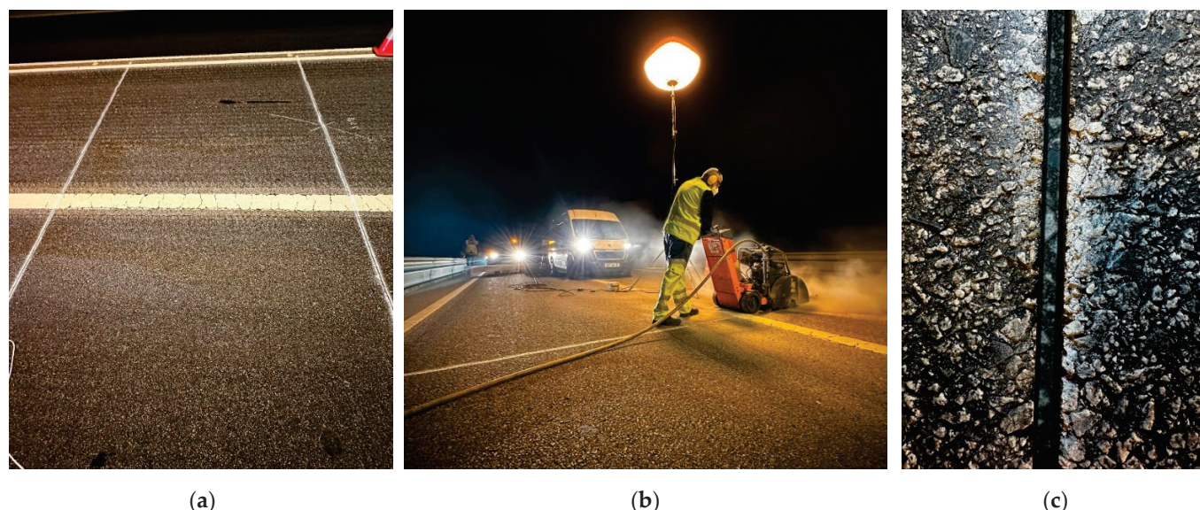
Figure 6. Initial phases of the pavement monitoring system installation: (a) markings for the precise positioning of the system; (b) the process of cutting the grooves; (c) visual inspection of one of the grooves.
