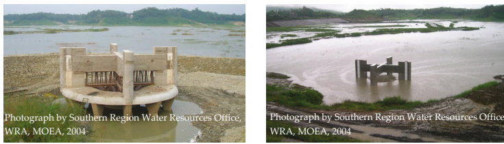
Figure 2. Shaft spillway pipe.
