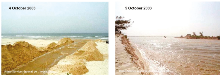
Figure 8. Ground photographs showing the initial trench (4 October 2003), dug on the night of 3 October 2003, across the Languede Barbarie to alleviate flooding of parts of St. Louis. The 5 October 2003 photograph shows the trench considerably widened by river and tidal flow (Photo credit: Service régional de l’Hydraulique, St. Louis du Sénégal).
