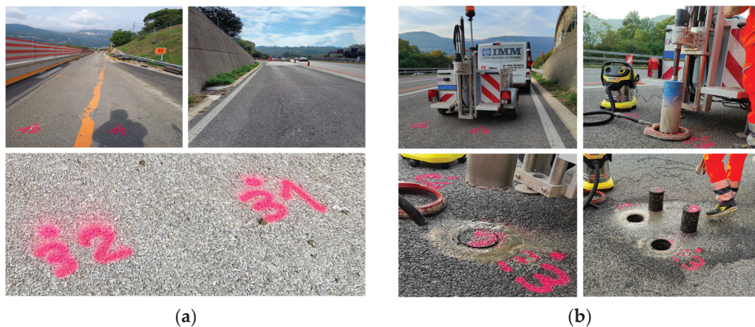
Figure 8. (a) Site inspection and coring points identification; (b) sample core drilling.
