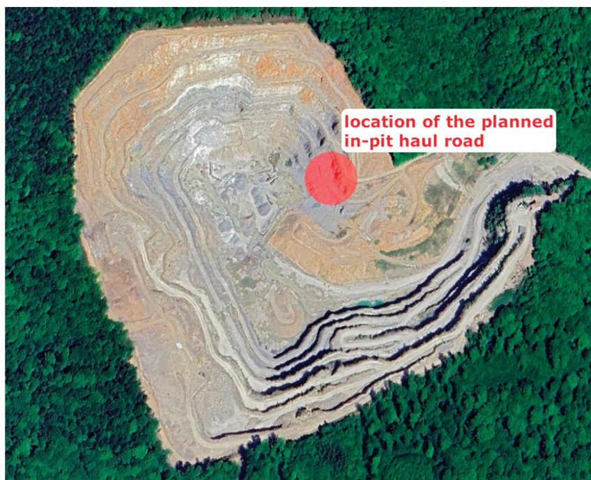
Figure 1. The location of the planned in-pit haul road in Dubie open-pit dolomite mine (source: https://www.google.com/maps , access date: 1 October 2025).
