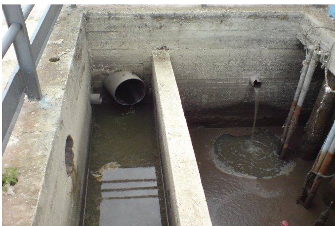
Figure 11. Close-up view of the sludge morphology before sonification. The non-uniform distribution of the particles and the presence of lumps indicate a slightly disintegrated state with a high tendency to sedimentation.
