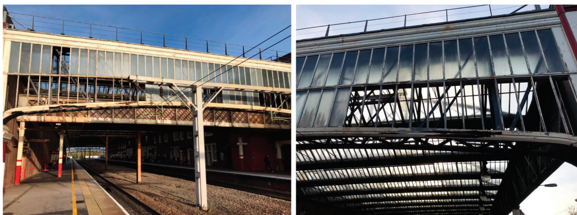
Figure 10. Condition of Stoke-on-Trent station gable ends before commencement of the replacement.
