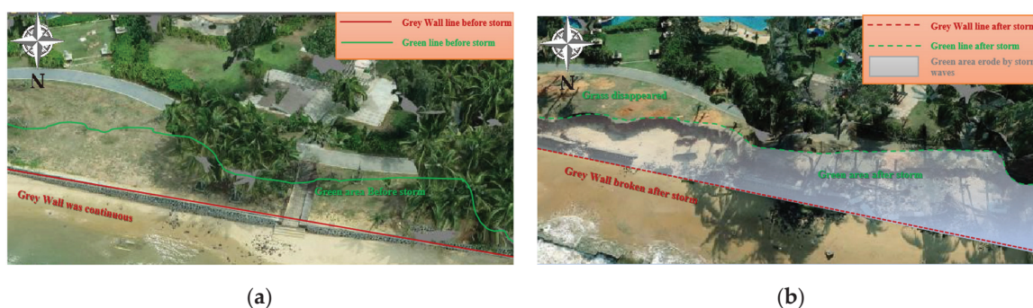
Figure 11. Beach berm with concert wall before (a) and after storm (b) in 2020 in Haikou Bay shows minor damage due to “grey method” by storm waves.
