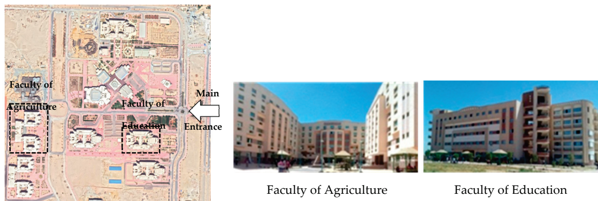
Figure 1. Satellite image and outside view of the two faculties in New Sohag University.
