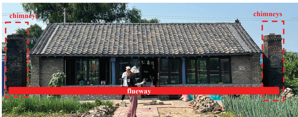
Figure 3. Typical Sibe traditional dwelling structure in Shifosi Village.
