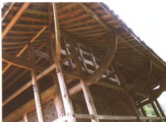
Figure 20. Complex corner structures and cantilevered elements in Tujia architecture (image source: Sun Yan).
