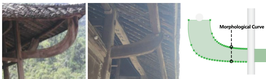
Figure 21. Morphology and simulation of ox-horn cantilevers.
