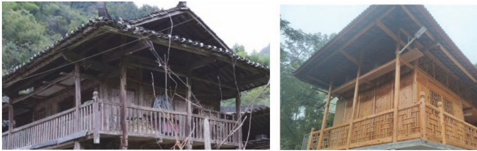
Figure 18. Complex corner structures and cantilevered elements in Tujia architecture.
