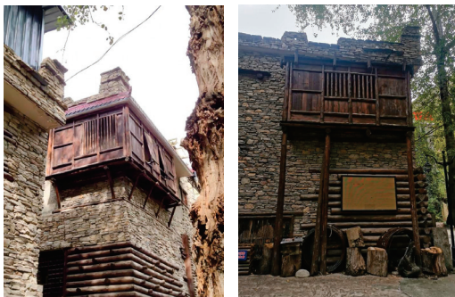
Figure 4. Actual photograph of the overhanging floors.
