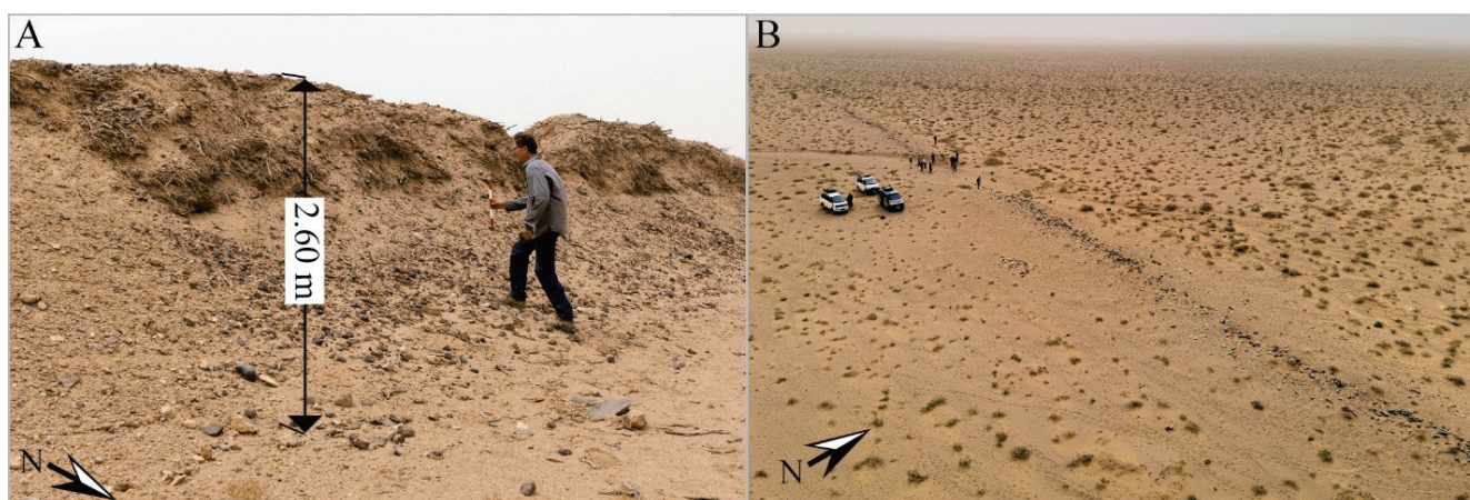
Figure 5. Wall sections. (A) Wall section between G03 and G04 the highest wall section. (B) Deteriorated wall section near G07 (Height up to 0.5 m) revealing the stones used.
