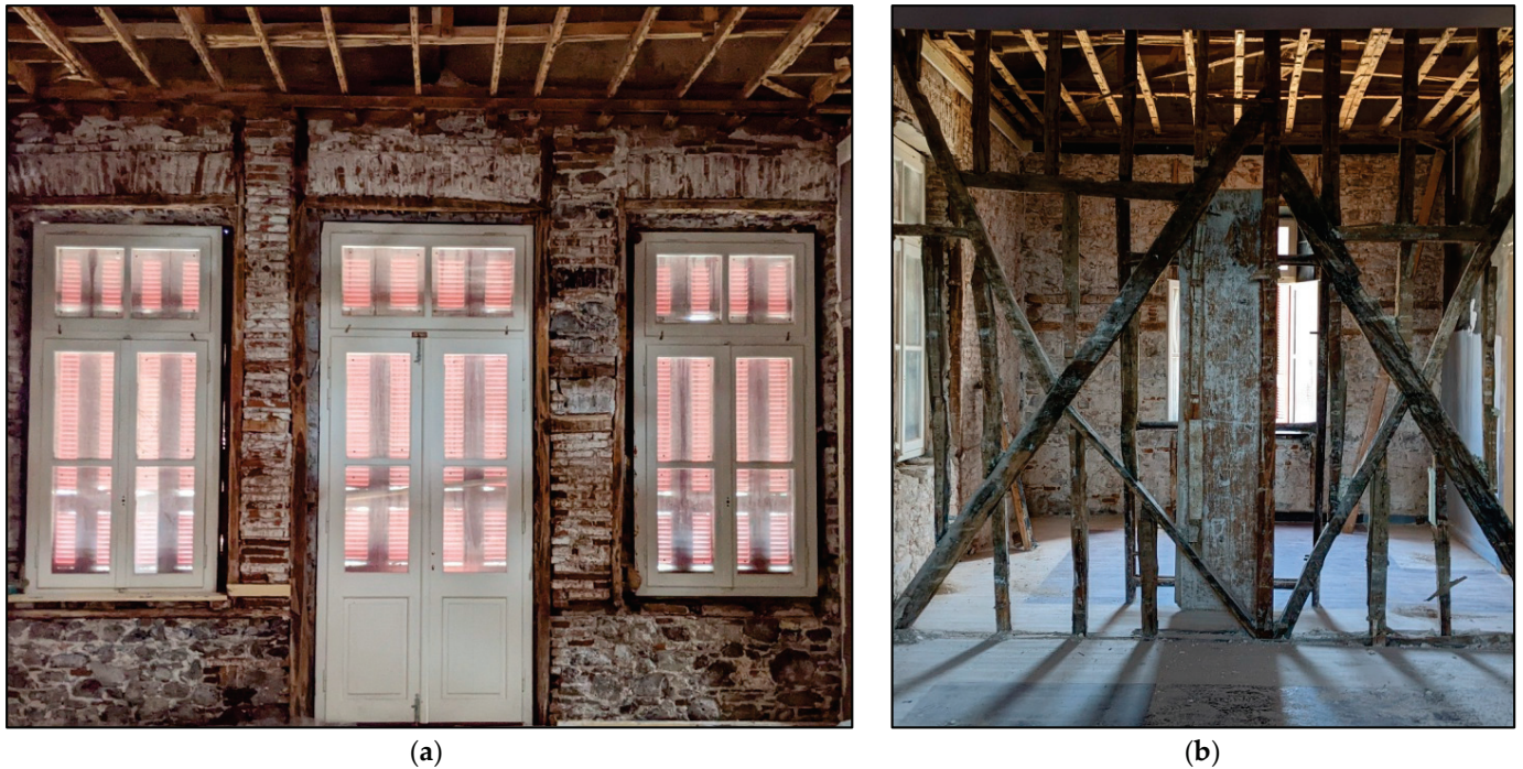
Figure 7. Structural features of the AML building at 2nd level: (a) Interior view of the external wall; (b) Baghdati internal wall. (Source: Digital Archive of the Ephorate of Antiquities of Lesvos, Hellenic Ministry of Culture and Sports; used with permission, Prot. No. 252765/16-06-2025).
