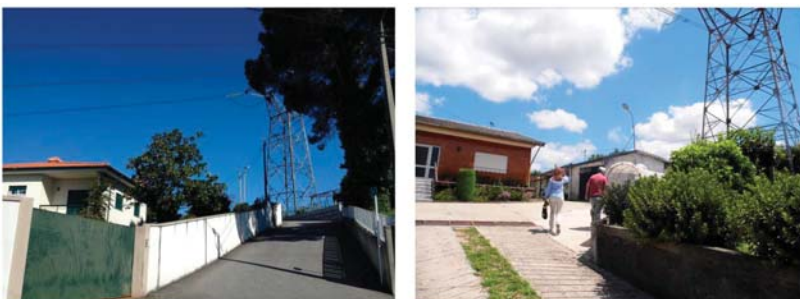
Figure 2. Power poles and power lines in the village of Serzedelo.
