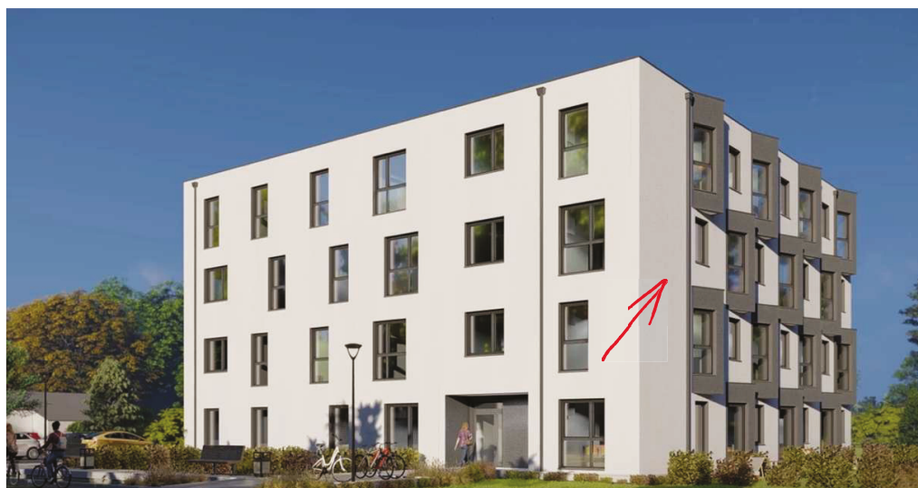
Figure 1. Modular building structure in the analysed case; the arrow indicates the location of the wall-mounted panels [38].
