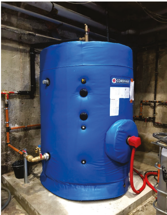
Figure 1. Regulated water temperature for concrete mixing in precast factory.
