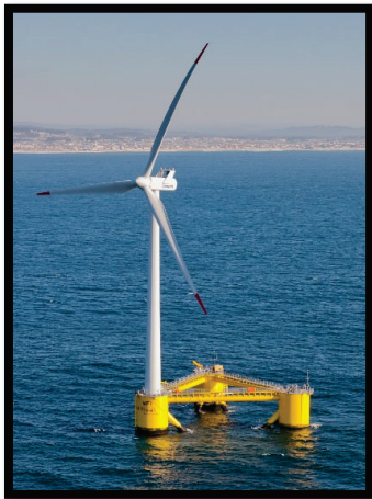
Figure 1. Offshore wind turbine with floating base [5].
