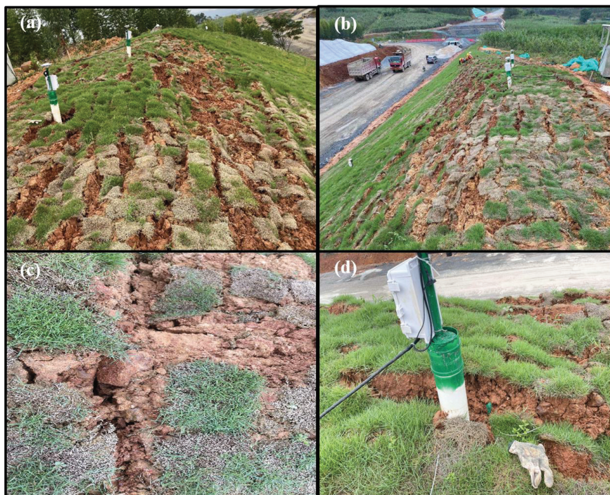
Figure 4. Shallow instability characteristics of Ningming expansive soil. (a–d) The visible cracks near the monitoring station.
