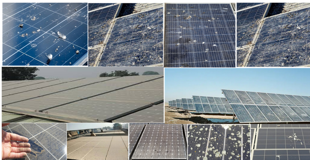
Figure 2. Various types of dirt and birds waste found on solar panels.
