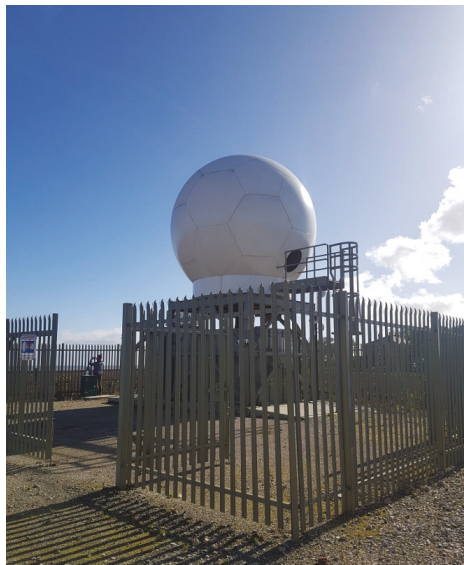
Figure 2. Doppler radar unit deployed on the shore of the Westermost Rough wind farm.
