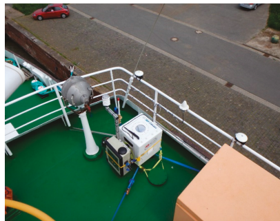
Figure 2. Installation of ship lidar System on deck of a medium-size vessel—© Fraunhofer IWES.
