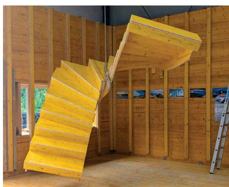
Figure 3. Wooden formwork for a conventional winder staircase.
