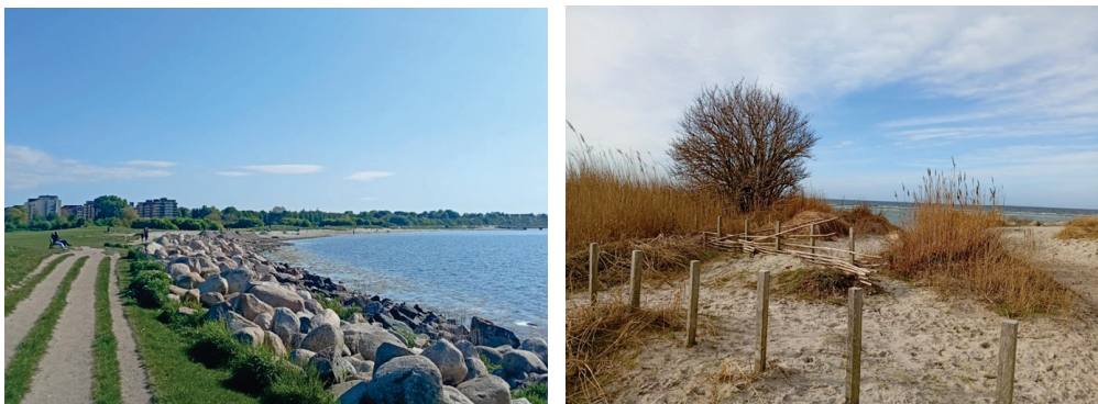
Figure 1. Examples of coastal management interventions in southern Sweden: (left) hard protection using rock revetments in the Malmö region; (right) soft, nature-based dune stabilization in Lomma.
