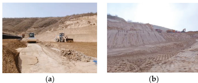
Figure 2. On-site subgrade construction. (a) Subgrade compaction; (b) terrain.
