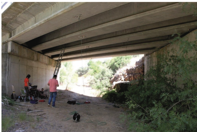
Figure 4. Arroyo Bracea I bridge (39°28′19.18″ N 3°49′48.39″ W).
