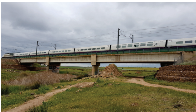
Figure 1. HSL bridge over Jabalón River ( 38^\circ 53' 51.3'' N 3^\circ 57' 53.0'' W).
