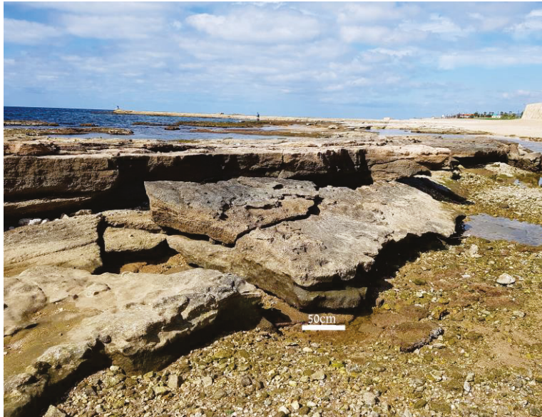
Figure 13. Blocks of beachrock outcrop under coastal, landward erosion north of Akko (Israeli coast), looking north (E. Galili).
