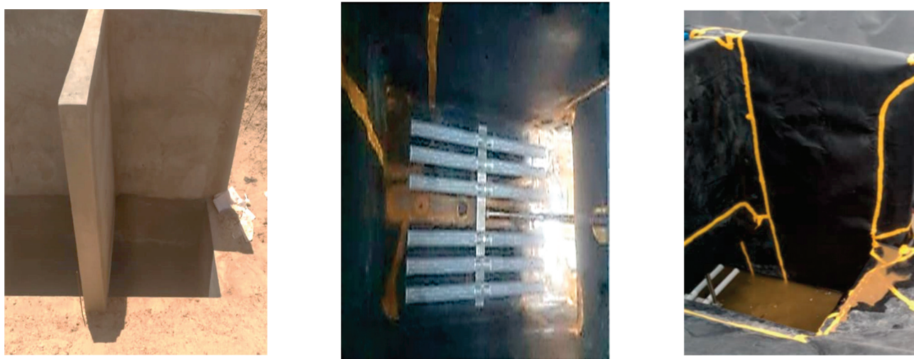
Figure 2. Photos of the Oxylag pit with air diffusers.
