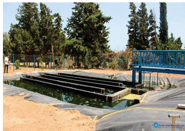
Figure 1. Photograph of ISA-CM combined Oxylag and High rate algal pond wastewater treatment demonstration pilot plant (COHRAP/WWTDPP).
