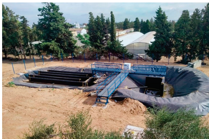
Figure 1. Photograph of ISA-CM combined Oxylag and High rate algal pond wastewater treatment demonstration pilot plant (COHRAP/WWTDPP).
