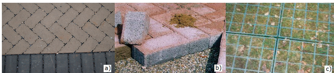
Figure 2. (a) Impermeable concrete PCIP (permeable concrete interlocking pavers); (b) porous concrete PCIPs; (c) grass-filled plastic grid pavers (PGPs).
