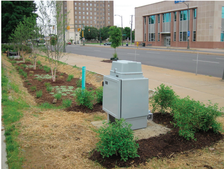
Figure 3. A bioretention facility at the Science Museum of Virginia in Richmond, Virginia.
