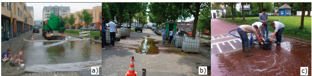
Figure 5. (a) Water truck supply; (b) water tank supply; (c) pumping from canal.
