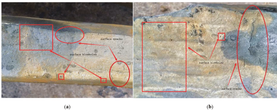
Figure 2. Surface cracks and blowholes on (a) web and (b) fillet of actual beam blank [5].
