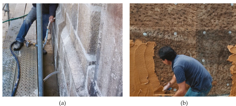
Figure 8. Examples of innovative strengthening solutions: (a) grout injection and (b) textile-reinforced mortar (TRM).
