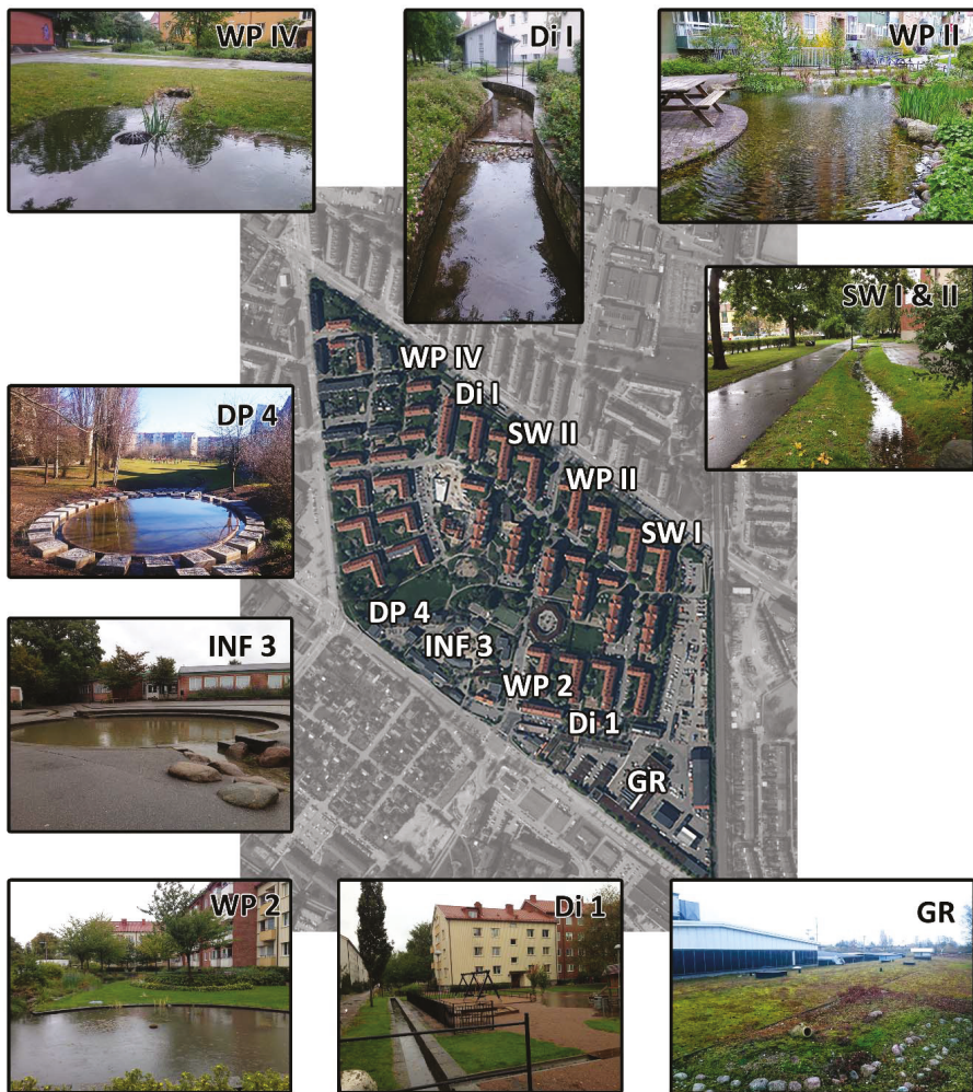
Figure A1. The photos of some of the implemented SCMs in Augustenborg. Different types of SCMs are shown in the figure as follows: (DP 4) dry pond, (Di I & 1) stormwater ditch, (SW I & II) swale, (WP 2, II & IV) wet pond, (INF 3) infiltration basin, (GR) green roof. The major runoff directions in the Northern and Southern systems are SW I → WP IV and GR → DP 4, respectively. Pictures for INF 3, WP 2, Di 1, and SW I & II are taken by Henrik Thorén (Rambøll). Background picture: GSD-Orthophoto, courtesy of The Swedish Mapping, Cadastral and Land Registration Authority, ©Lantmäteriet (2015).
