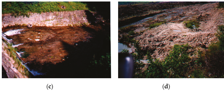
Figure 3. Mlynne stream—cross sections modified with check dam and water reservoir upstream of the check dam. (a) check-dam; (b) check-dam reservoir with coarse sediment; (c) down stream of a check-dam; (d) fine sediment in a check-dam reservoir.
