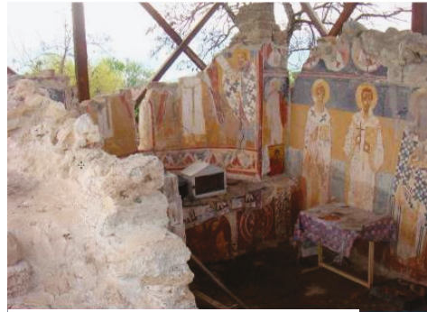
Damaged by the 1995 earthquake
