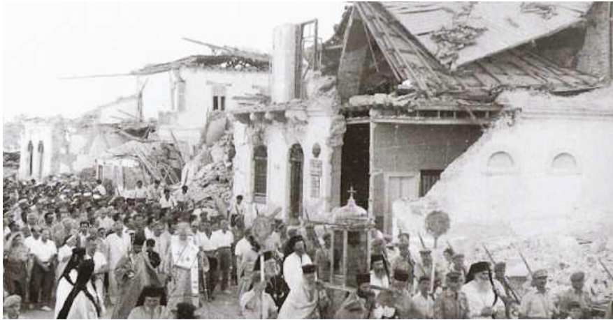
Figure 22. Images of total destruction to old masonry construction in Argostoli, Kefalonia island during the 1953 earthquake sequence.
