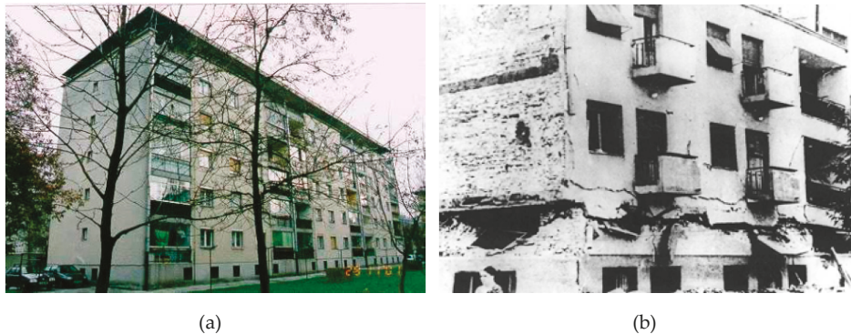
Figure 2. (a) Typical building in Slovenia; (b) devastation of a typical building after the 1963 Skopje earthquake [4].
