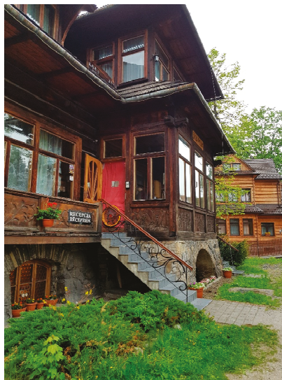
Figure 6. Tightness test at the ‘Stara Polana’ hostel (authors’ own image).
