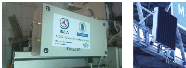
Figure 2. Relay RSU (left) and installation of Sending RSU on a variable message panel (right).
