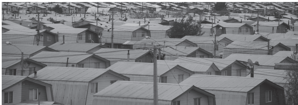
Figure 1. Social housing development in Los Angeles, southern Chile.
