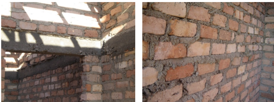
Figure 9. Excessive use of mortar increases the environmental damage as well as the overall construction costs. Source: The authors.
