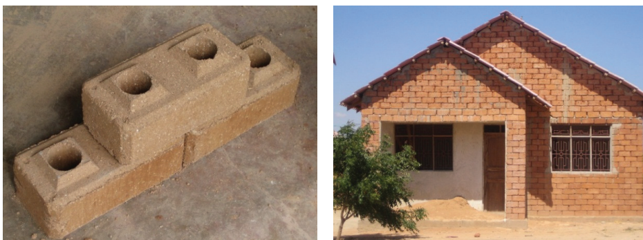
Figure 10. Interlocking bricks can be an alternative for burned bricks. Source: The authors.
