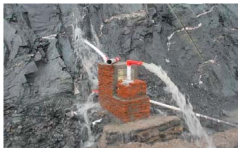
Figure 11. Pipe draining of rainwater and groundwater away from Nanfen open-pit mine slope.
