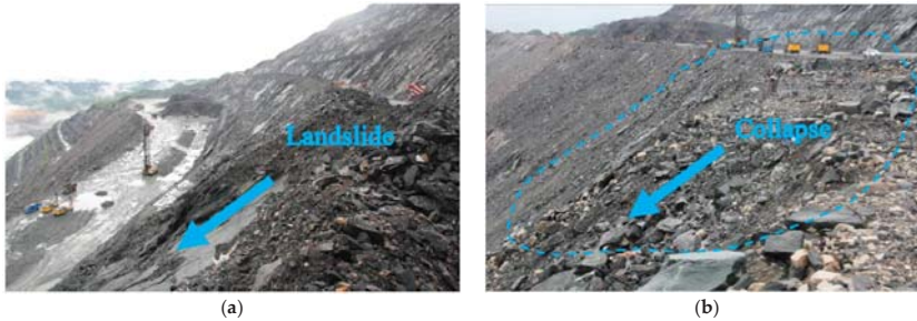
Figure 1. Landslides and collapses caused by rainfall. (a) local landslide; and (b) overall collapse
