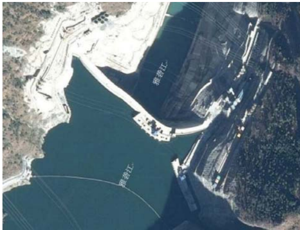
Figure 1. A bird's eye view of Jinping I Hydropower Station by man-made satellite.
