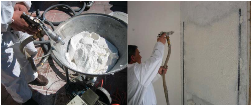
Figure 2. In situ application of the aerogel-based plaster.
