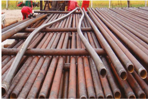
Figure 3. Excessive bending of the inner tubing at a Chinese salt cavern storage [3].
