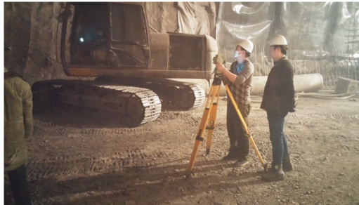
Figure 27. Total station measurement.
