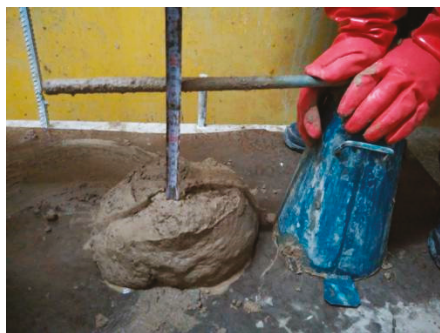
Figure 2. Slump test at the construction site.
