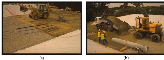
Figure 12. Placement of (a) one of the pipe series in the gneiss sections, and (b) the 500-mm concrete pipe.
