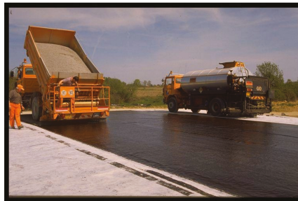
Figure 5. Placement of the 3-layer asphalt wearing.
