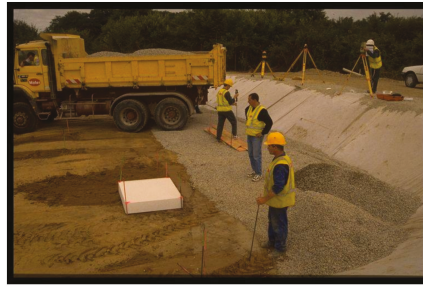
Figure 7. Placement of one of the polystyrene blocks in the silt section.
