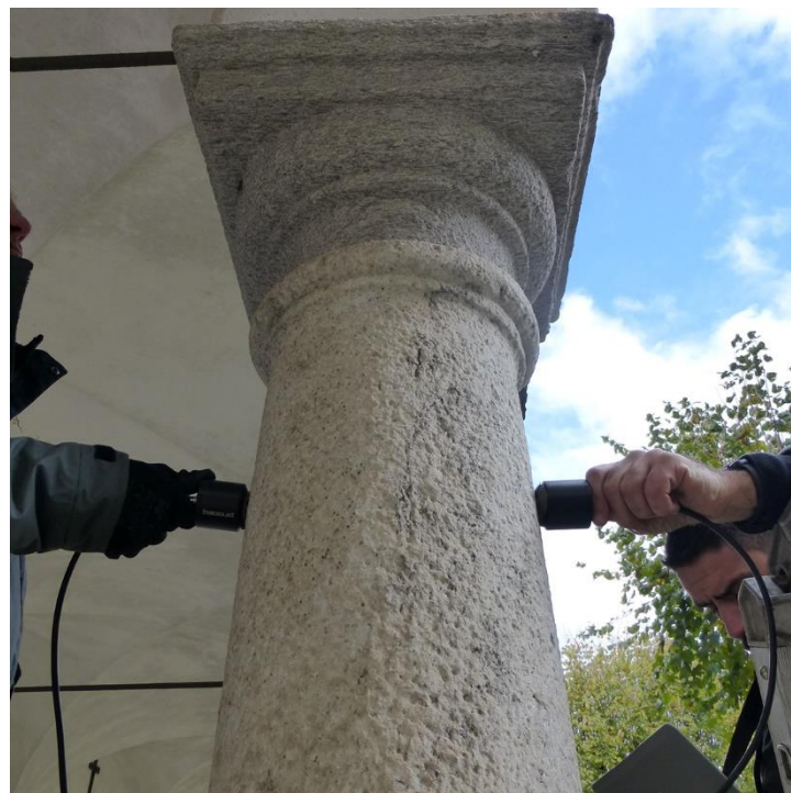
Figure 4. Ultrasonic test carried out on columns of Via Crucis, Ghiffa.
