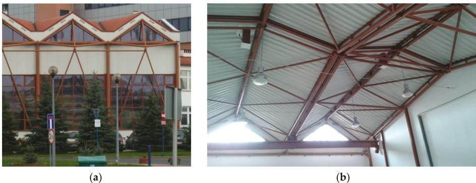
**Figure 1.** A roof shell structure composed of many transformed fold shell strips: (a) view from the outside; (b) view from the inside.
