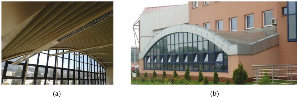
**Figure 6.** A transformed roof shell whose inside bottom layer is folded sheeting: (a) view from the inside; (b) view from the outside.
