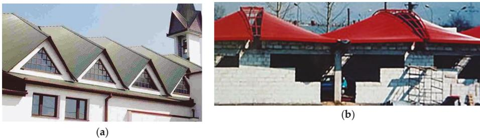
**Figure 2.** Two shell roof structures characterized by: (a) two straight directrices; (b) straight and curved directrices.
