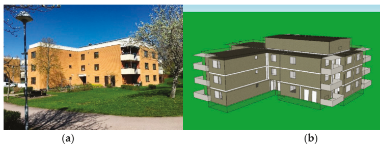
Figure 1. (a) Building that was modeled. (b) Model of the building in IDA-ICE (IDA Indoor Climate and Energy).
