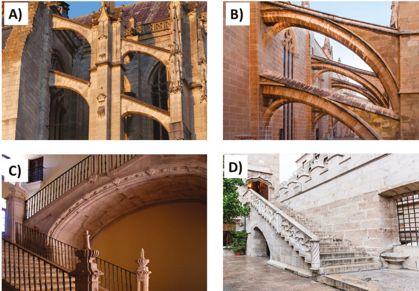
Figure 3. (A) One- and two-arch circumference flying buttresses of Beauvais Cathedral (France). (B) Flying buttresses of the Cathedral of Palma de Mallorca. (C) Rampant arch in the staircase of the Monastery of Uclés (Cuenca). (D) Rampant arch in the staircase of La Lonja (Valencia).
