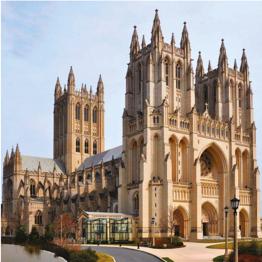
Figure 4. Washington cathedral and its flying buttresses.
