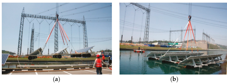
Figure 13. Lifting and launching process; (a) Lifting; (b) Launching.
