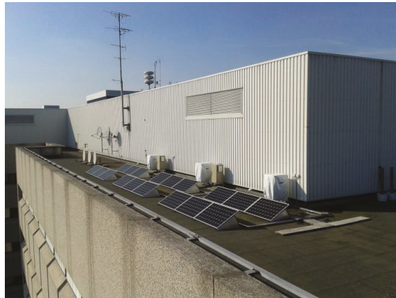
Figure 5. The experimental facility of SEAC.
