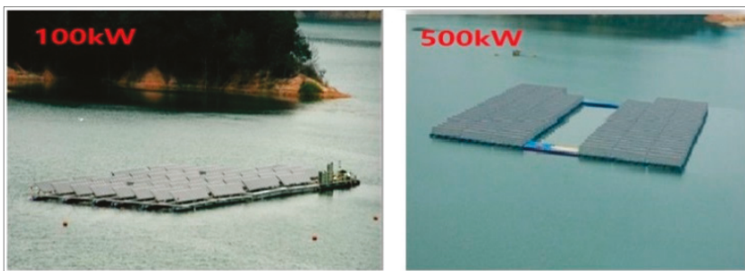
Figure 1. Aerial view of the 100 kW (left) and 500 kW (right) floating systems on Hapcheon lake.
