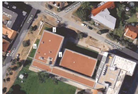
Figure 11. Measuring points outside the building (Source: https://www.google.com/maps/place/Debrecen ).
